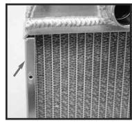
PHOTO 3: Folded over radiator side channel.
